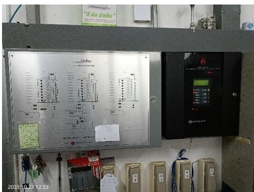
Fire Alarm Control Panel : FCP
